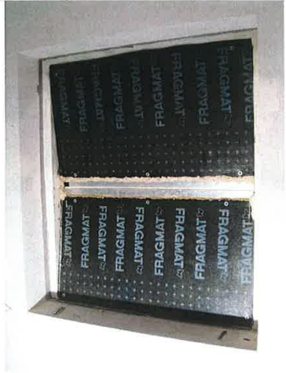
Test opening during measuring (Laboratory 2 – receiver room)
