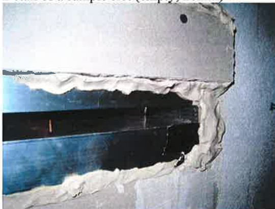
Photo No. 24299d-05
