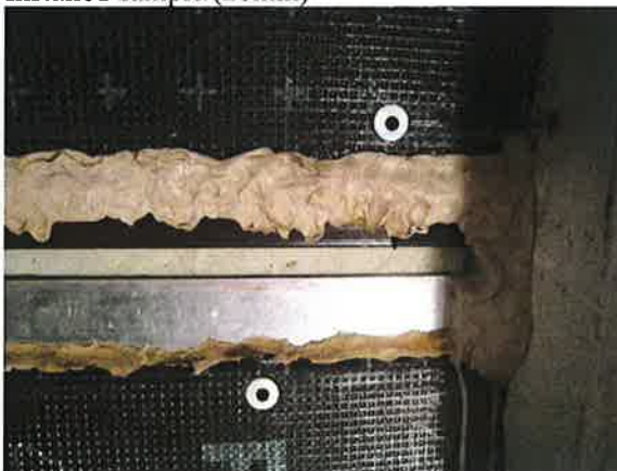
Photo No. 24514d-10
